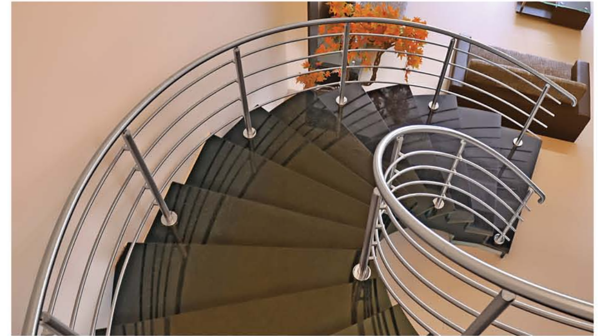
Top Mounted Round Baluster System with Horizontal Members - Ø 38/50mm (DT11-1-164)
